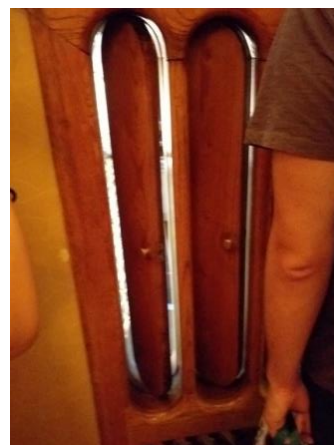
Figures 5 and 6 - Biomimetic example of a ventilation model inspired by the work of fish gills, in the house of Batlló - an overview and explanation of the ideas and functions of this model is given through a virtual tour (Augmented and Virtual Reality)
