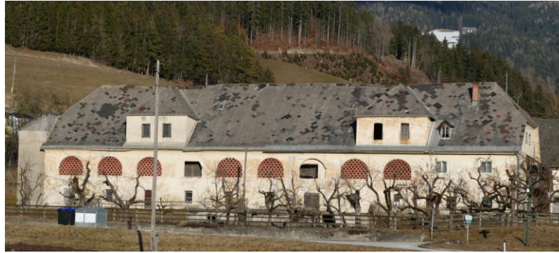
Figure 24 - Combined stable and barn with later adaptations, showing symmetry and lattice-work of bricks in ist wall openings. (Klein St. Paul, Austria; photo G.Weiss 2016)
