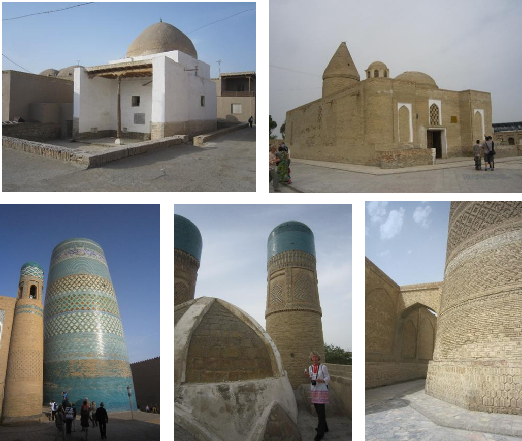
Figure 21 - Medieval vaults and towers in Khiva and Bukhara (Uzbekistan) with ornamentation by brickwork and glazed ceramic tiles (photos G. Weiss 2014)
