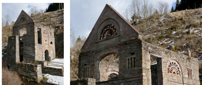
Figure 25 - Ruin of a furnace from the 19th century in Lölling, Austria. It shows rosette decorations made of bricks similar to barn decoration. (photo G.Weiss 2016).
