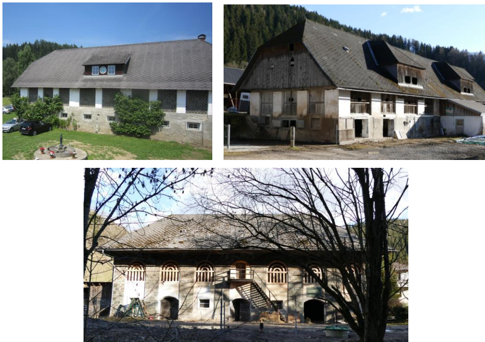
Figure 23 - Typical Carinthian combined stable and barn buildings showing module structure as well as overall symmetry (Carinthia, Austria. Fotos G. Weiss 2015)
